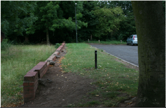
Perimeter wall along Swanslength
